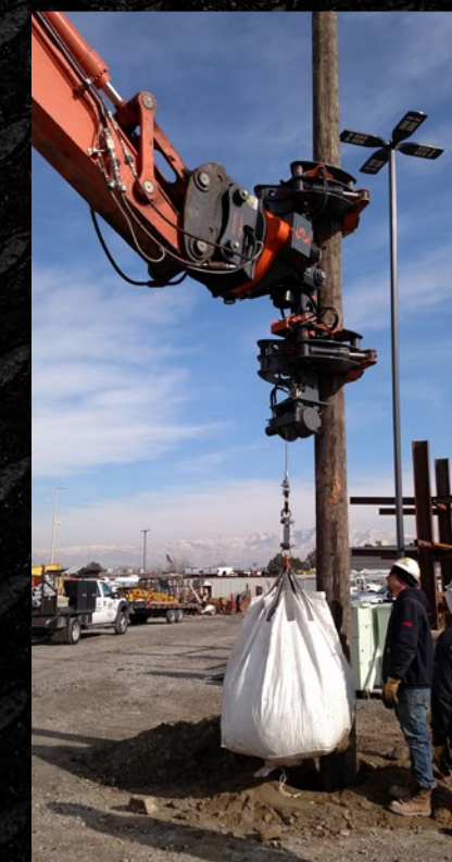
Utility Winch for Pole Setting
